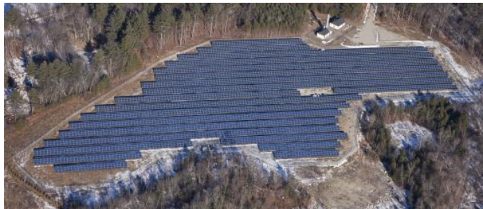
Photo of the 1.72 MW array at the Grafton Water District
