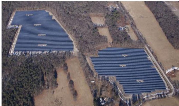
Photo of the 4.8 MW and 3.6 MW arrays in Franklin, MA
