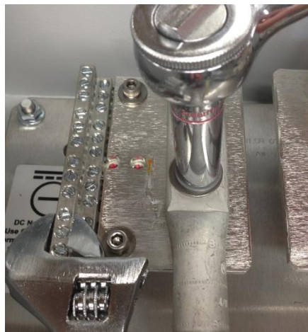
Picture 2 – Crimp Lug Option with Backup Wrench
