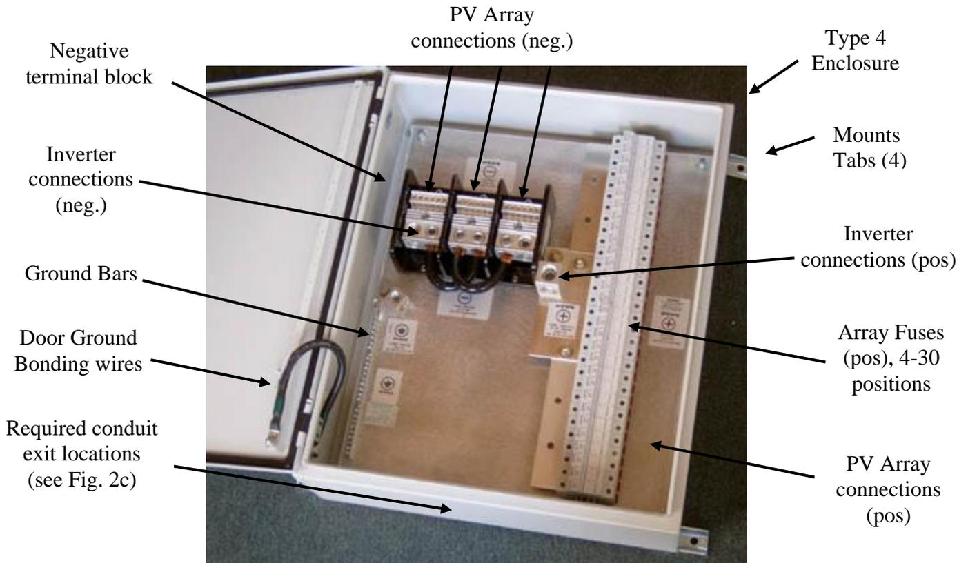
**Fig. 4 Fused String Combiner Features and Connections**
