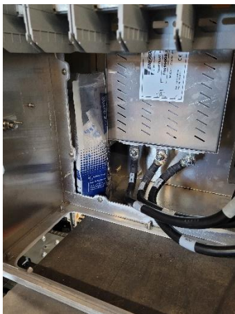
Figure 3-19 Proper Location and Orientation Options for the Desiccant Pack
