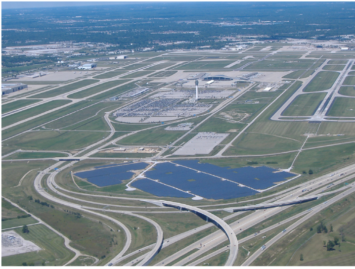
Project: Indianapolis Airport Solar Farm • Location: Indianapolis, IN System Size: 10MW • Installer: Cenergy • Product: (20) SGI 500XT
