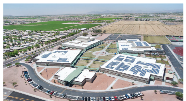
Project: Campo Verde High School • Location: Gilbert, AZ System Size: 400kW • Installer: Solar City • Product: (4) PVI 82 KW
