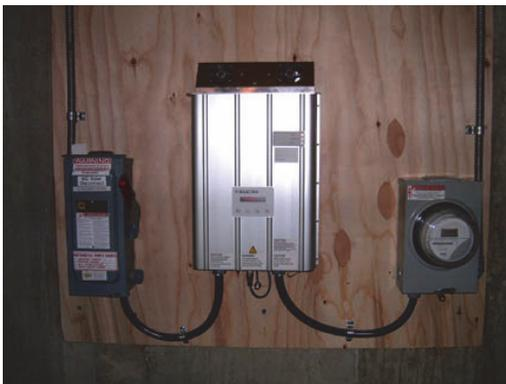
Typical mounting on plywood board (Sunlight Solar)
