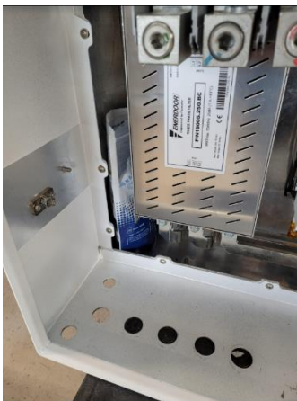
Figure 3-17 Proper Location and Orientation Options for the Desiccant Pack
