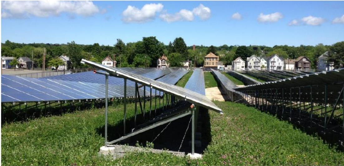
Figure 11. PV Panel Installation with different tilt angle at Haverhill site
