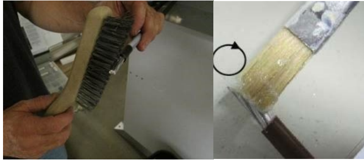
Figure 4-38 Preparing Aluminum Wires Prior to Connecting
